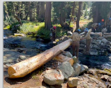
Constructing a durable log bridge buttressed with granite slabs & boulders.
